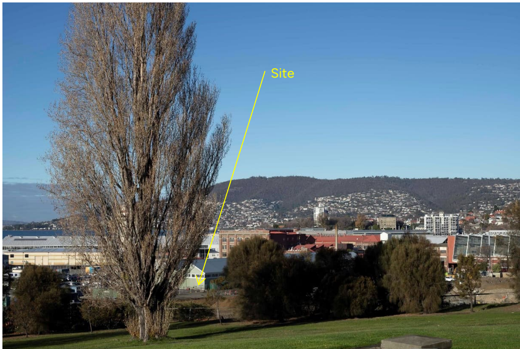
Figure 9 View to the south into the Site from The Cenotaph
