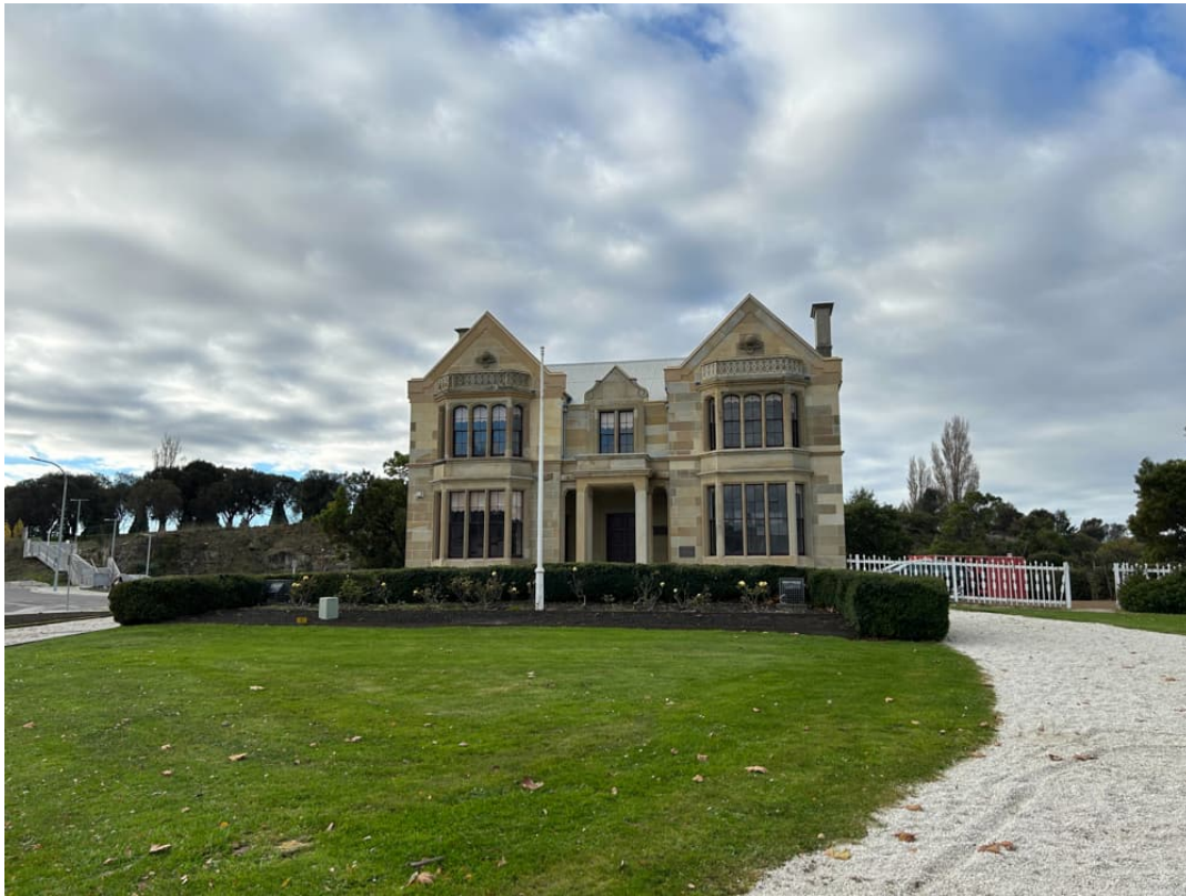
Figure 3 Royal Engineers Building on the western edge of the Site
