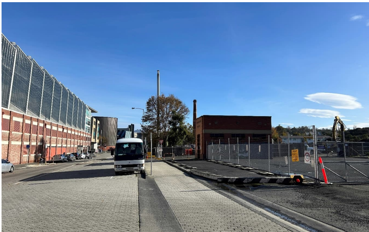
Figure 16 Views to the northwest along Evans Street
