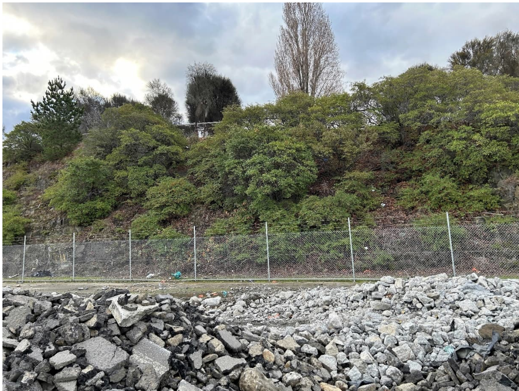
Figure 7 Vegetated Escarpment along northern boundary of the Site
