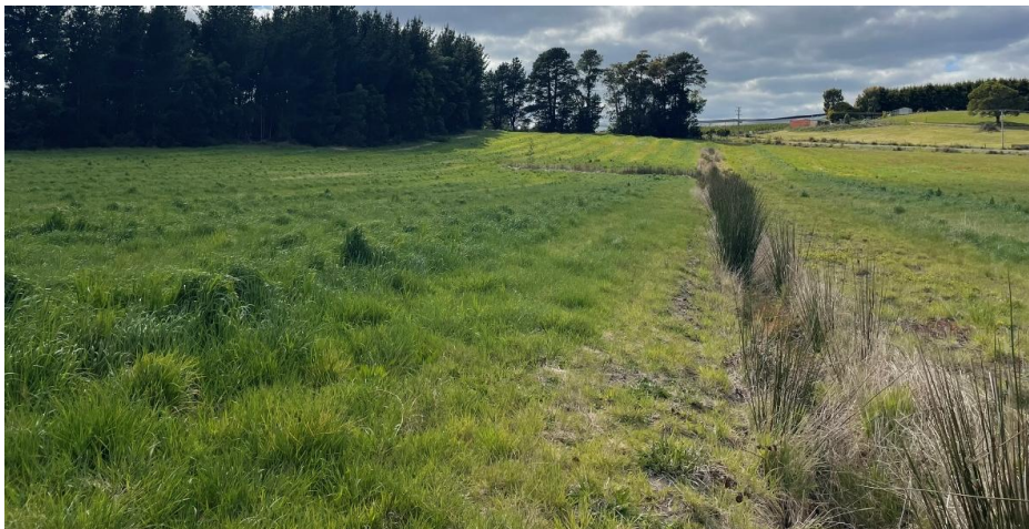
Figure 8 Existing man-made drain on site
