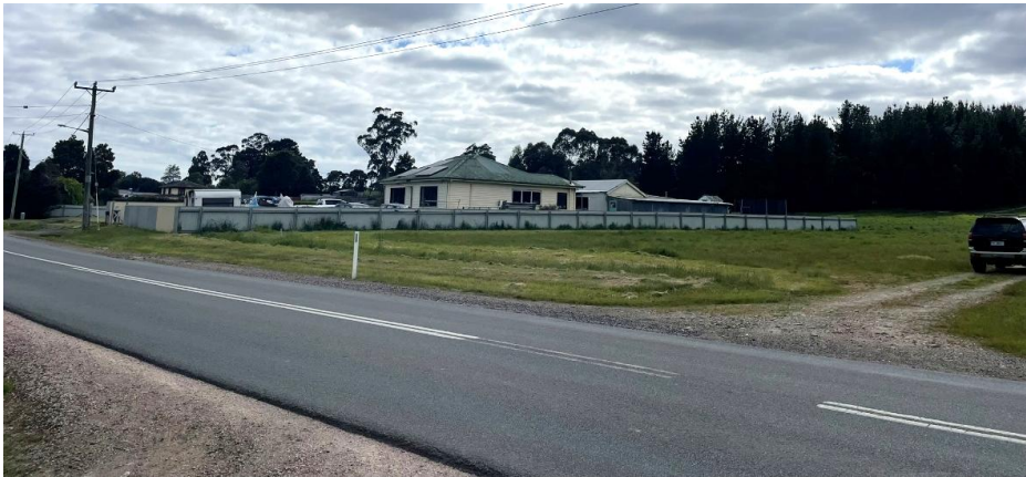
Figure 6 Adjoining dwelling (229 Sheffield Road), existing access from Sheffield Road.
