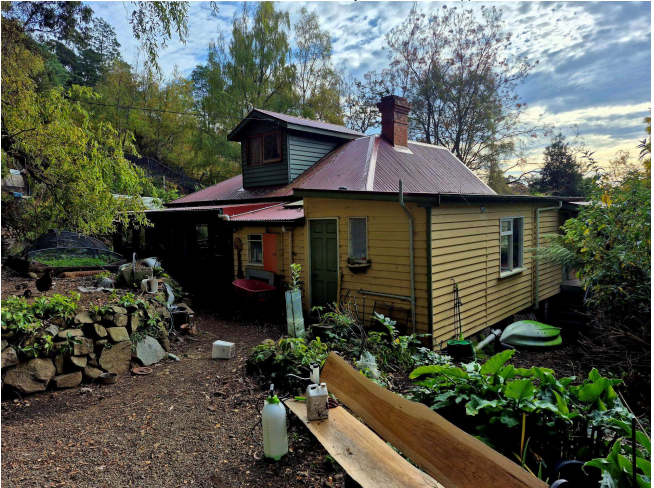
Photo 1 below – 3 bedroom two bathroom residence recently renovated and approved western view
