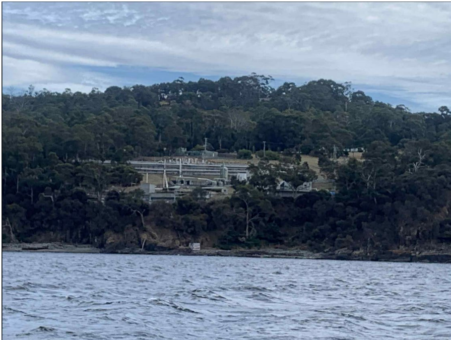
Figure 4: Photo from the East, water side looking toward the subject site. Note the Tas Water Treatment Plant dominating the view/landscape. Top A. Shows Water Treatment Plant, built in ~1990s, refurbished ~2016/2017. Bottom B. shows Water Treatment Plant with expansion of infrastructure (a water pump station to service the Golf Course) on the high point approved ~2019 and photographed 2026, in alignment with my dwelling in elevation. It should be noted that I objected to both of these developments and other's objected, even having the objections heard at TASCAT. Both the initial development and expansion were approved through State and Local Government mechanisms. See Annexure B for details on the development of this Plant and extensions.
