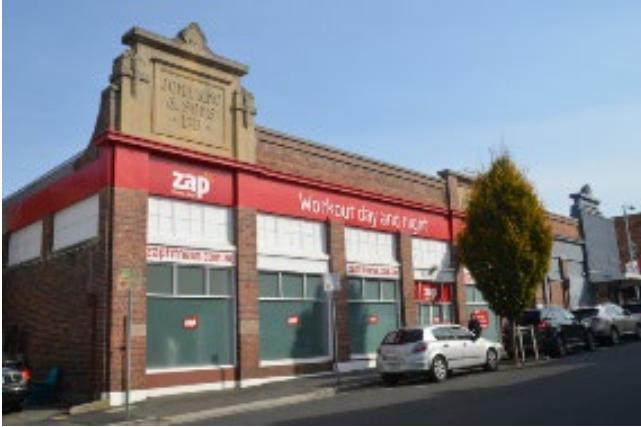
Figure 3 - Intact facades on adjoining title - No.2 Kingsway
