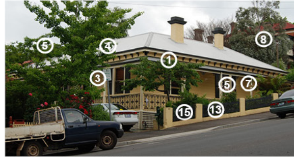
37 Lawrence street - Mid Victorian single dwelling
