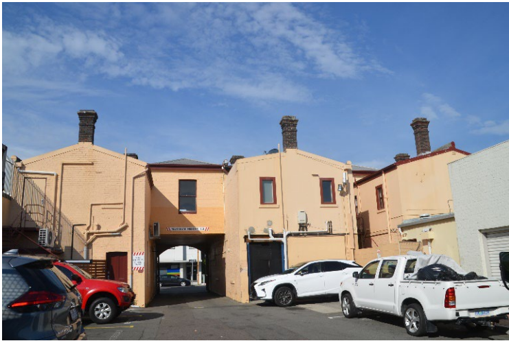
Figure 2 - Rear of the Building (192 and carriageway at left)
