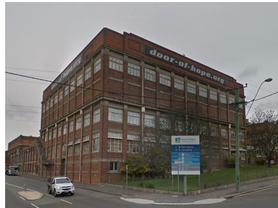
Figure 1 (from Google Street View)
