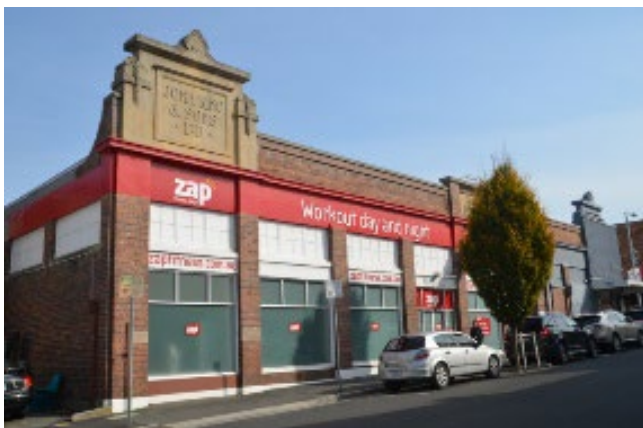
Figure 2 - Intact facades on adjoining title - No.2 Kingsway
