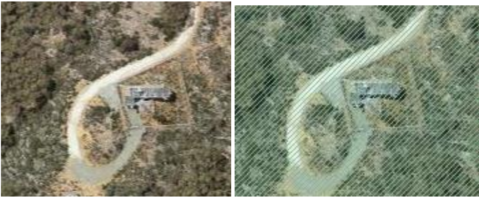
Figure 6 Priority Vegetation layer applied to Grey Mountain Communication Site
