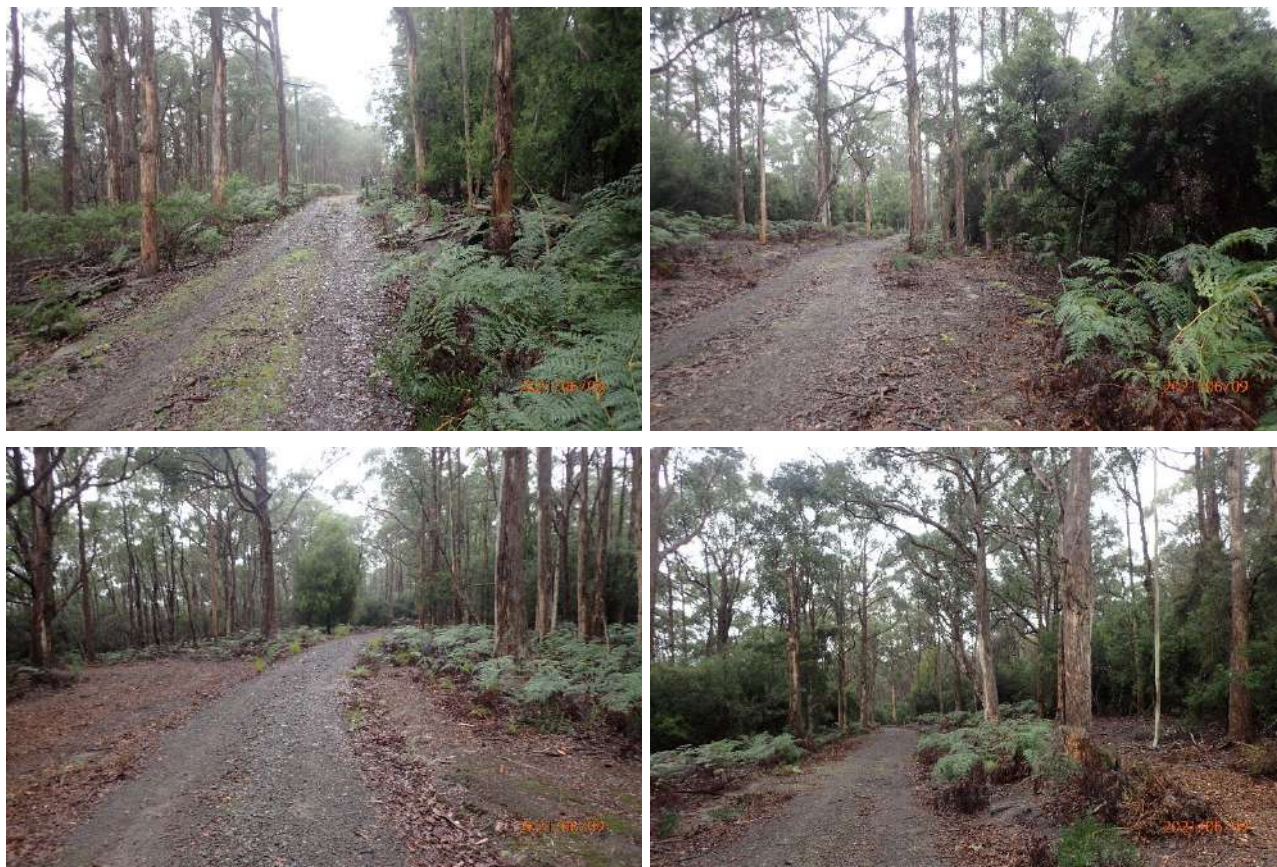
Plates 1-4. Existing access route including entrance gate, well-formed pavement, existing clear table drains and various opportunities for passing bays lacking native vegetation per se
