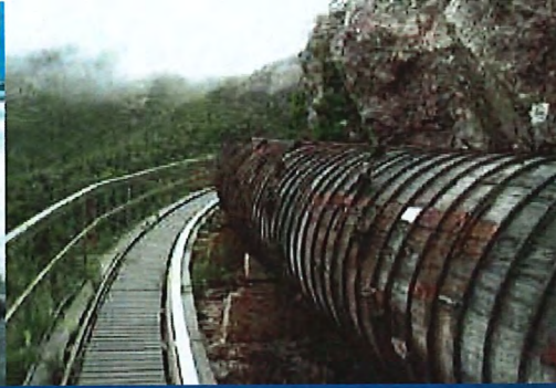
Left: The Lake Margaret Woodstave Pipeline on the west coast is part of Tasmania's historic heritage Heritage Tasmania
