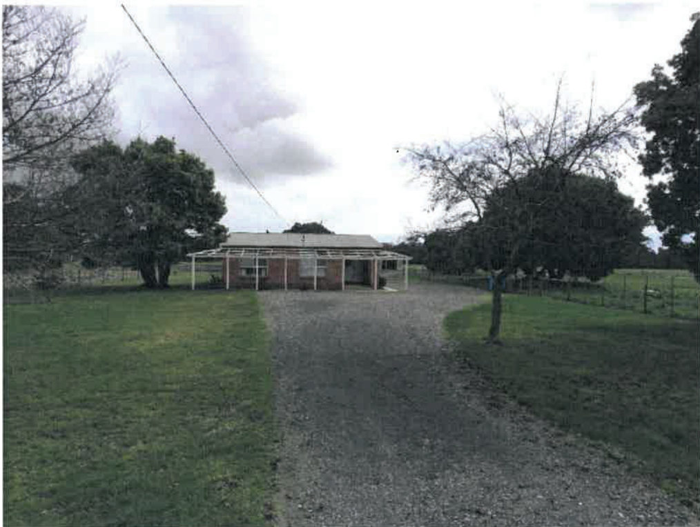
Figure 5; existing residential 2 bedroom dwelling on the far south east corner of the property
