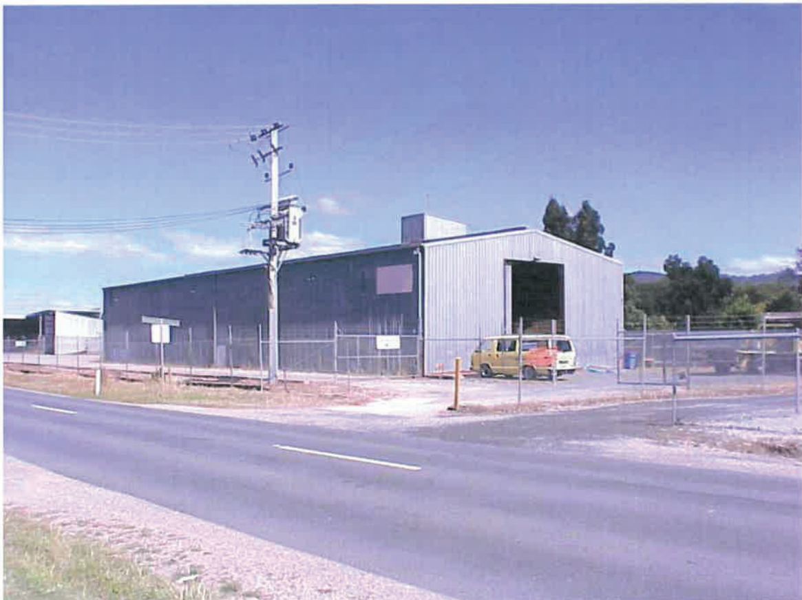
Photo looking south towards the main shed from Mersey Main Road
