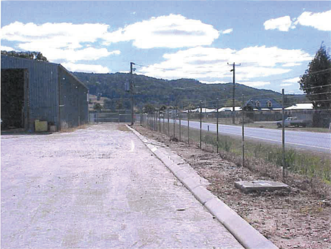
Photo looking north-west along the Mersey Main Road frontage.
