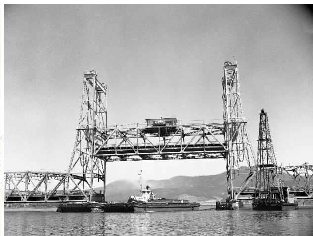
Figure 9 Bridgewater bridge – a vertical lift, Pratt truss through bridge. (Source: 'Tugboat with barges from APPM Boyer passing under the Bridgewater Elevator bridge', 1957, TAHO, AB71311/5575)
