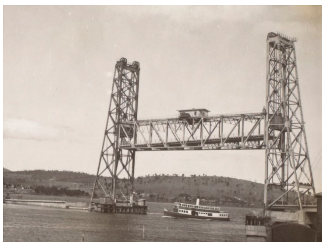
Figure 4 The floating Derwent Bridge, Hobart c1943 (Source: 'The first vessel through the lift span' , c1943, Agent-General's Office Album of Views, Libraries Tasmania)
