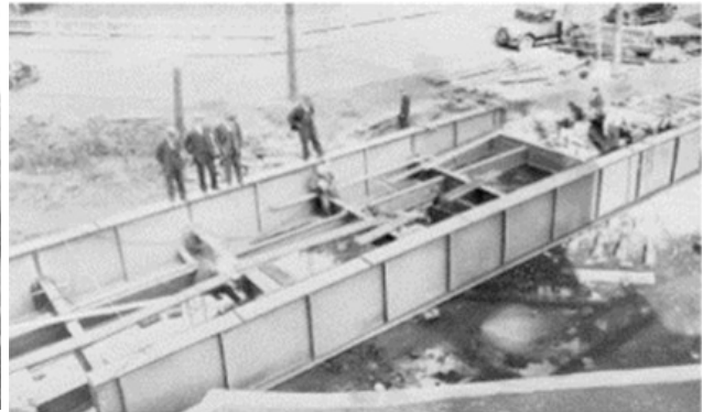
Figure 2 A 1930-1945 half through plate-girder deck bridge in Münster, Germany (Source: Alencar, et al, 'Fatigue cracking of welded railway bridges', p 157).
