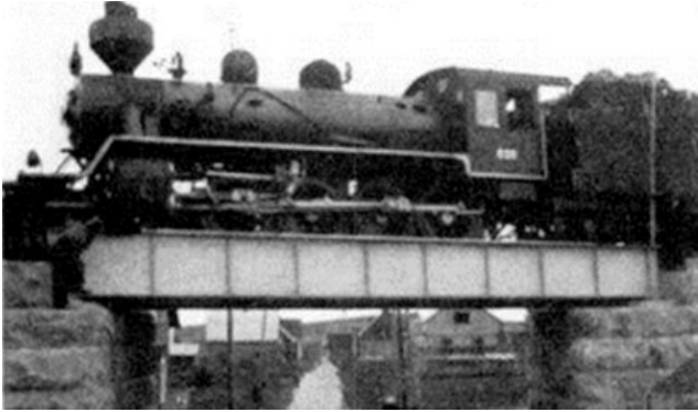
Figure 1 A c1933 plate-girder deck bridge, Helsinki, Finland (Source: Alencar, et al, 'Fatigue cracking of welded railway bridges', p 157).
