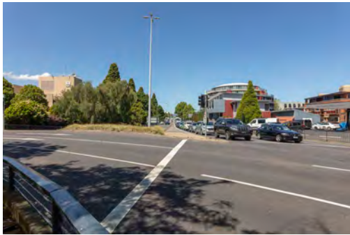
KOP 13 - RAILWAY ROUNDABOUT BROOKER AVENUE
