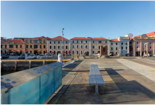
KOP 11 - VICTORIA DOCK BRIDGE
