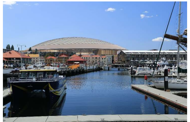
High pedestrian area of Elizabeth Street pier, in contrast to KOP 11 where the H. Jones buildings do not obscure the stadium.
