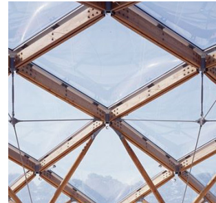
RT01 ETFE roof skin with hybrid steel and timber structure
