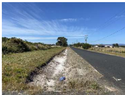
Figure 15 Site frontage to Arnold Street looking south southwest
