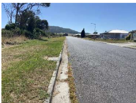
Figure 20 Site frontage to Stonehouse Street looking east
