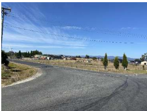
Figure 14 Road network Arnold Street and North Street looking south west
