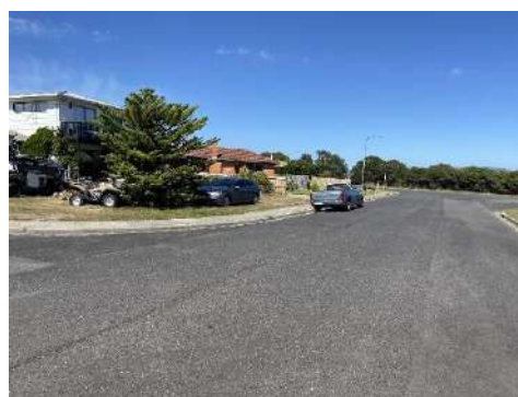
Figure 17 Surrounding residential development - Stonehouse Street looking west
