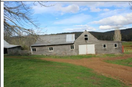
Figure 4: View of Shearing Shed from the West
