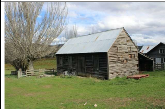
Figure 6: View of Barn from the North
