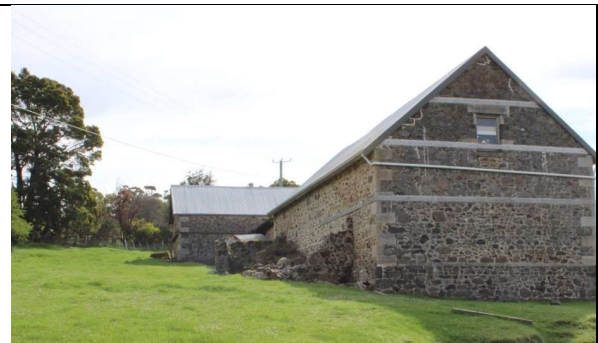
Figure 3: View of rear West façade of Stables building and annex
