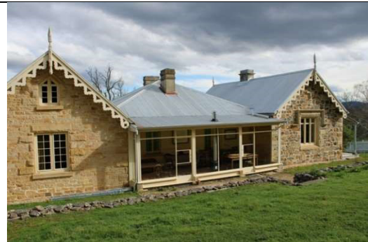
Figure 3: View of Farmhouse – rear façade
