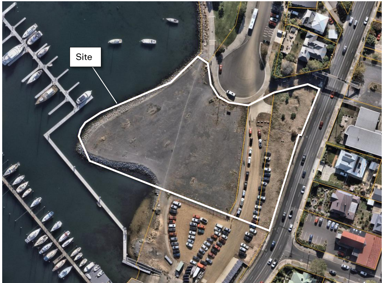
Figure 4-2: Existing Site Aerial Photograph
