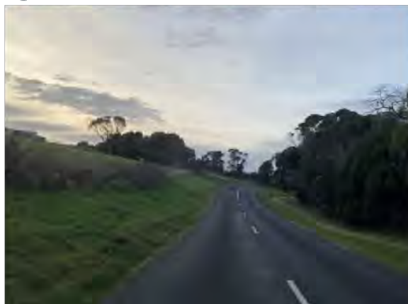
Figure 32 – Golf Links Road – Westbound from Table Cape Road.
