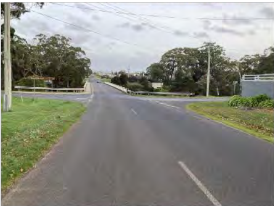
Figure 13 – Table Cape Road Northern approach to the junction.
