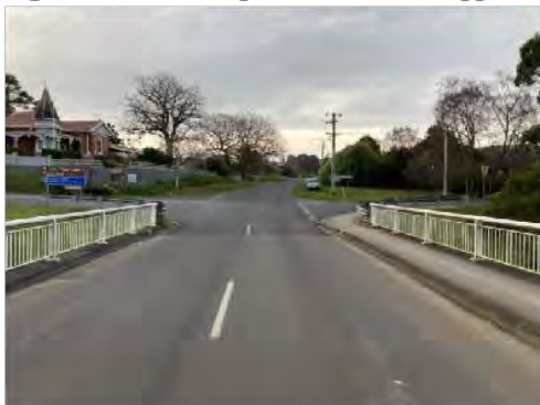
Figure 11 – Table Cape Road Southern approach to the junction.
