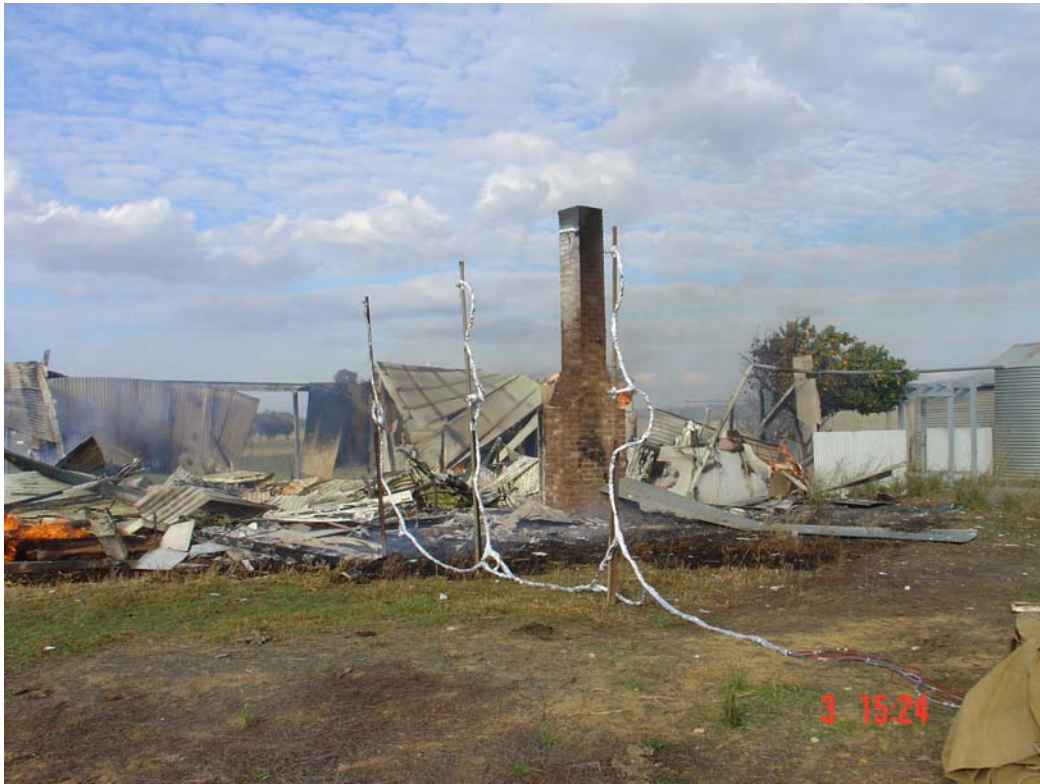
Figure B7. Aftermath of the fire
