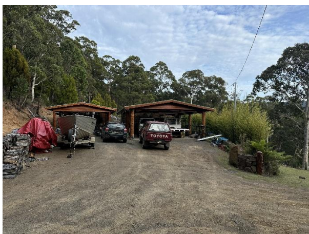
Fig.4 Driveway, shed and carports
