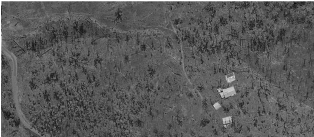
Figure 7. 1967 bushfire destruction – 18 Feb 1967
