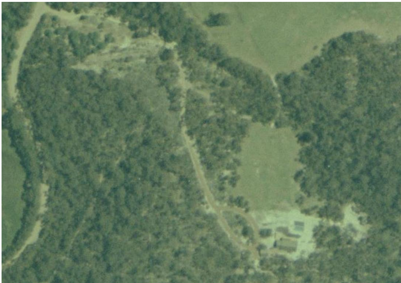
Figure 8 Newly completed house and ancillary structures – 13 Jan 1997
