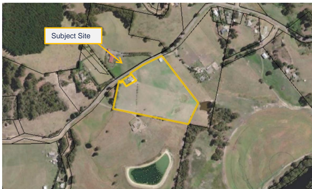
Figure 1 - Aerial view of the subject site (Source: LISTMap)
