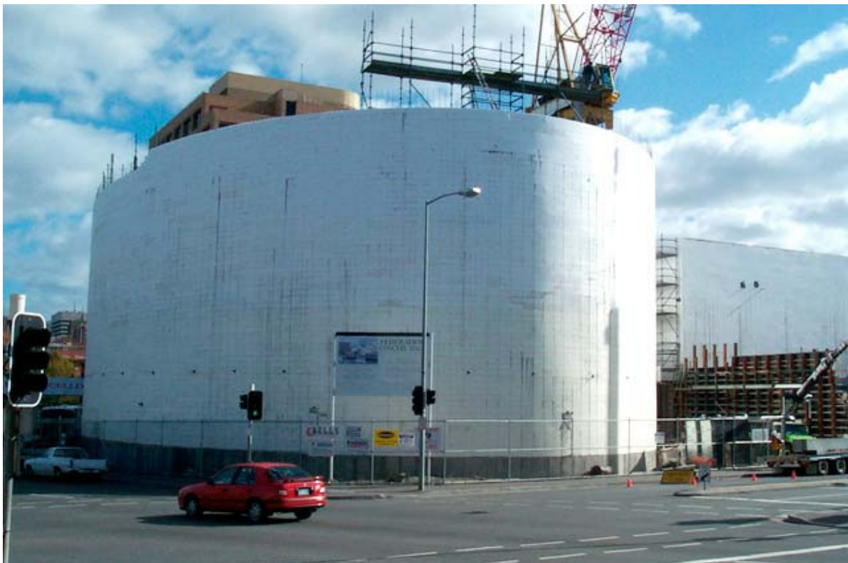
Figure 21-8 Construction image from "Thermacell"
