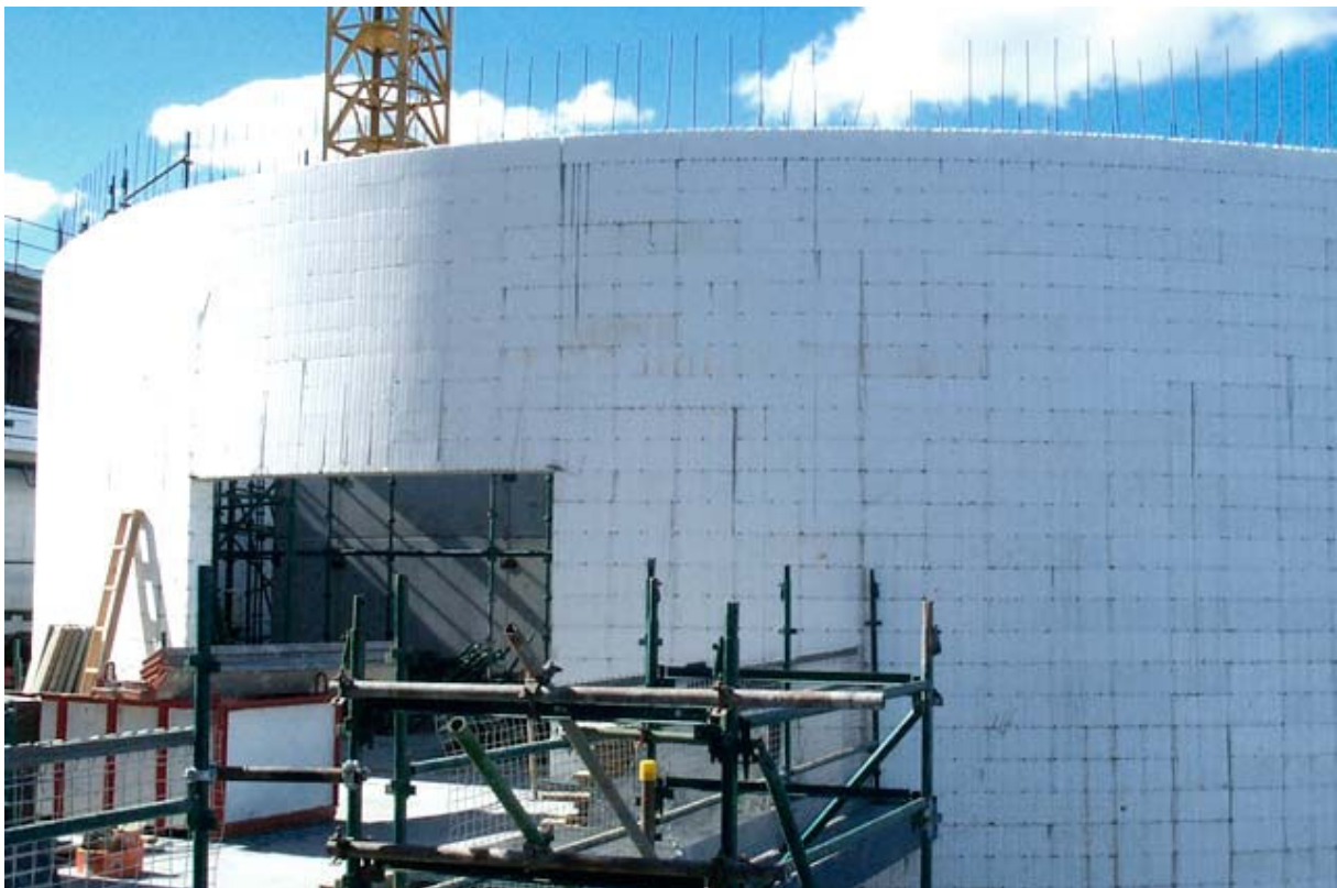
Figure 21-4 Construction image from "Thermacell"
