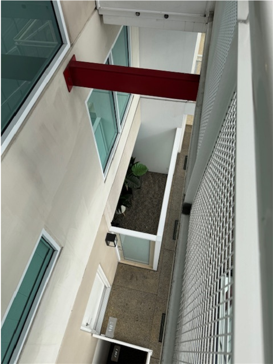
Figure 22-2 Fixed glazing within Sullivans Cove Apartments
