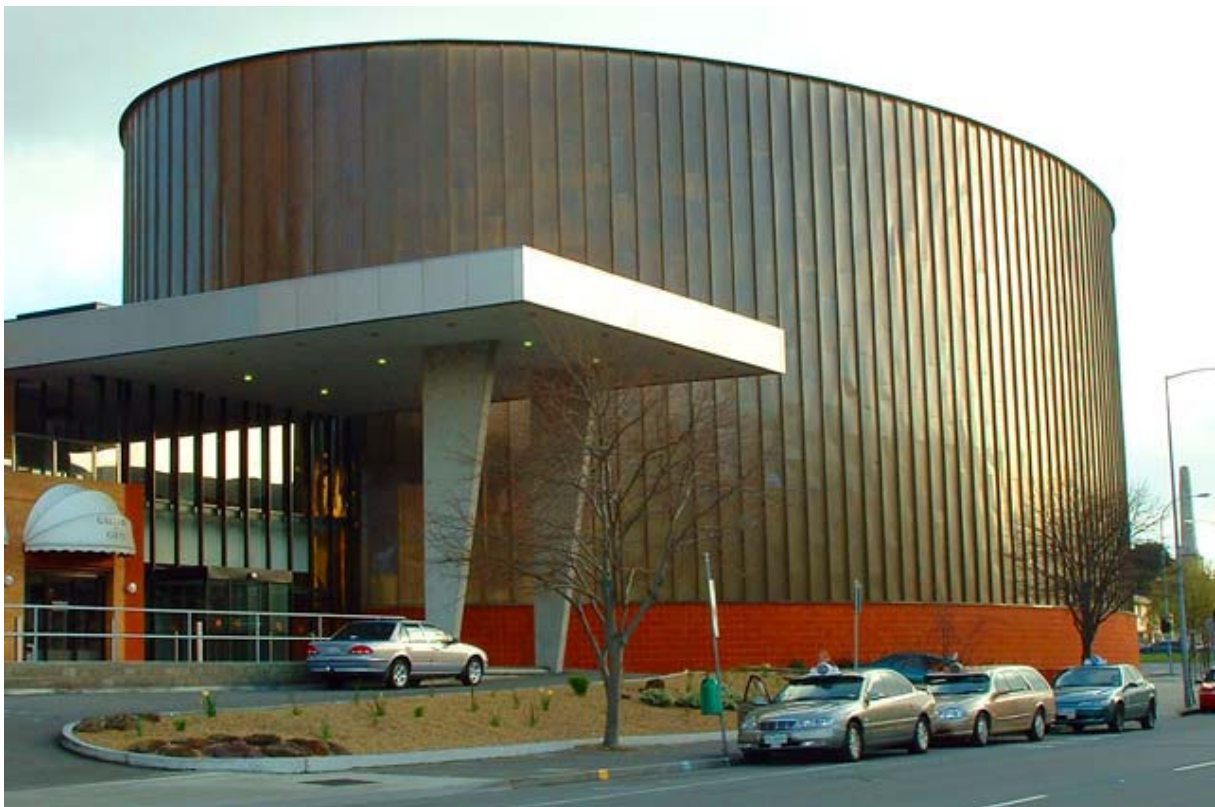
Figure 21-10 Construction image from "Thermacell"
