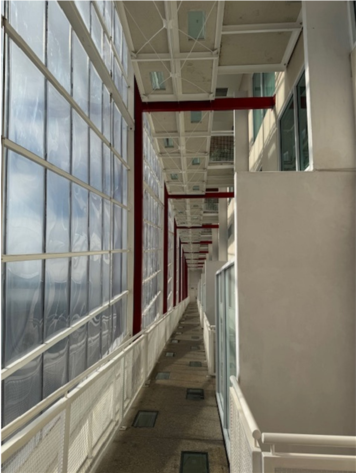
Figure 22-1 Secondary facade to Sullivans Cove Apartments
