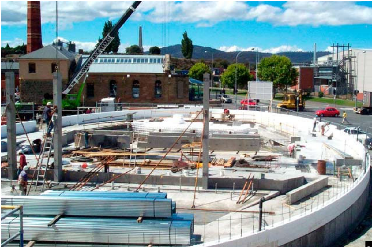
Figure 21-3 Construction image from "Thermacell"
