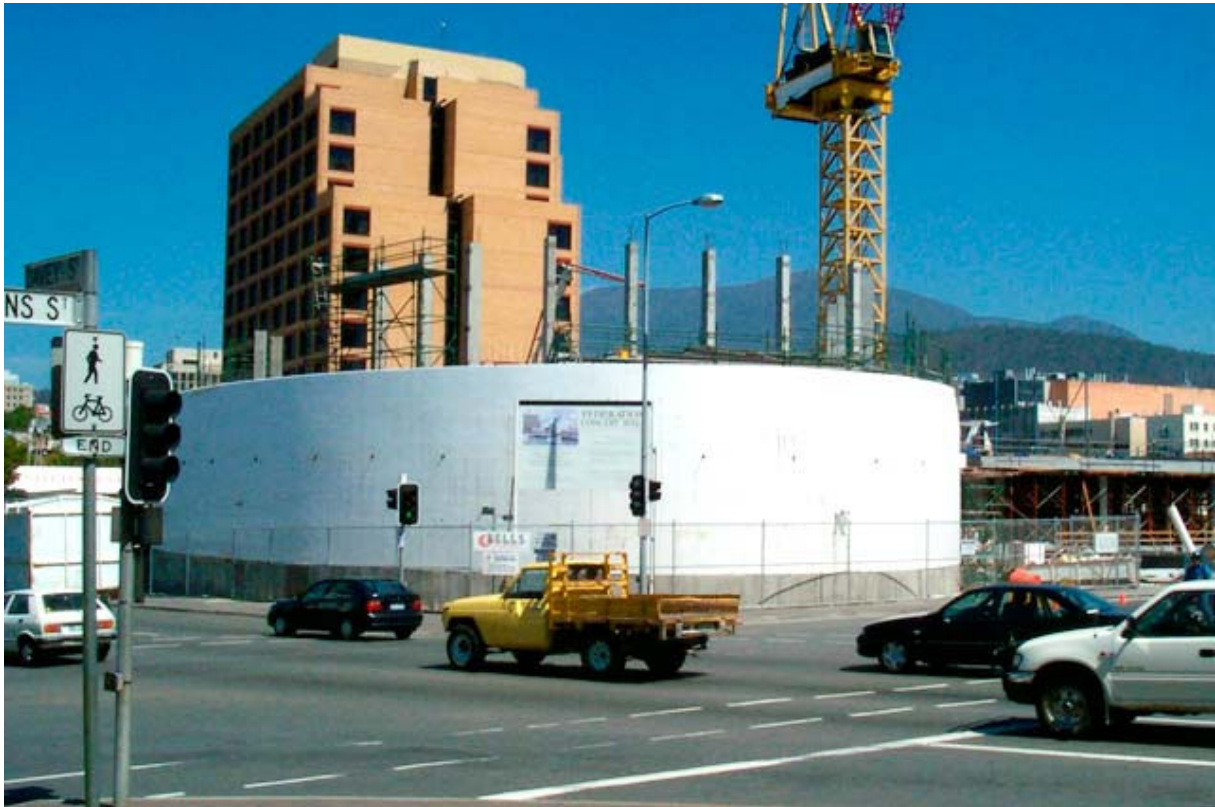
Figure 21-5 Construction image from "Thermacell"
