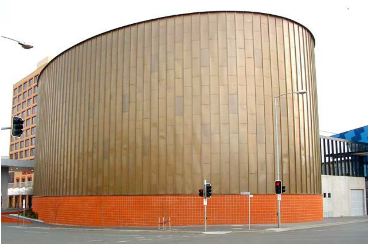
Figure 21-9 Construction image from "Thermacell"
