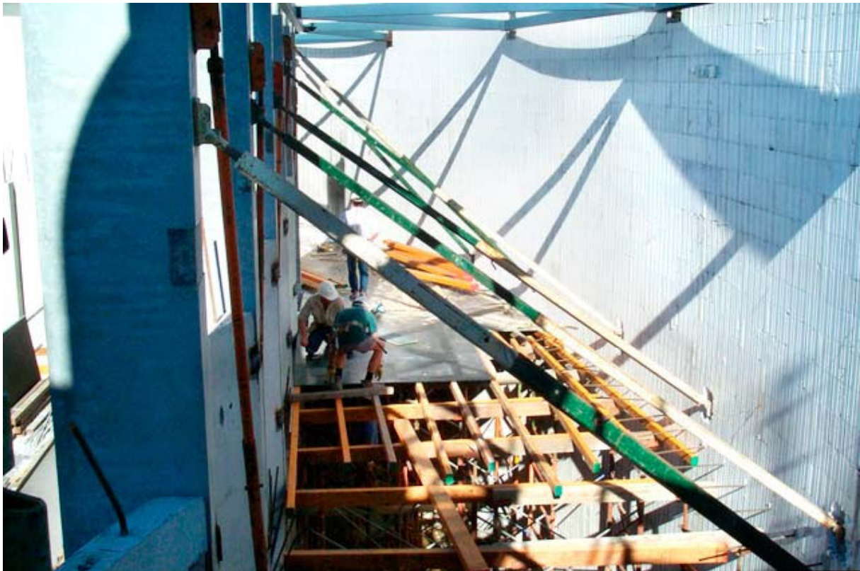
Figure 21-6 Construction image from "Thermacell"
