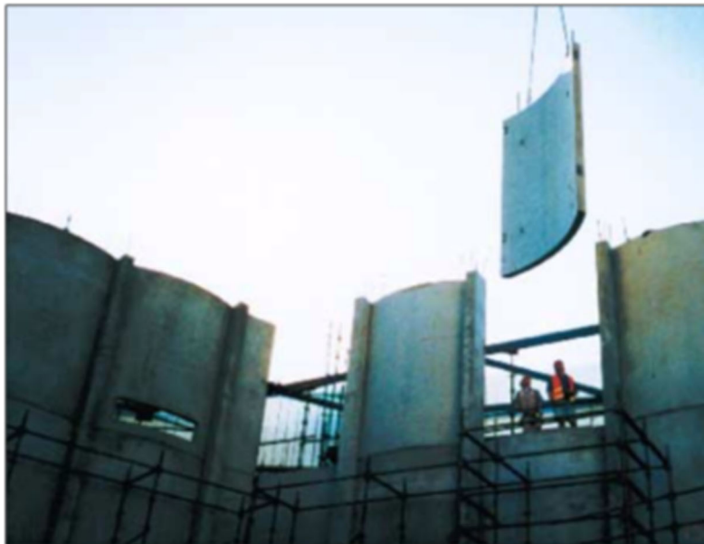
Erection of upper level precast blade columns (top) and erection of 4.1 m high curved panels which form auditorium's main interior walls (above).
