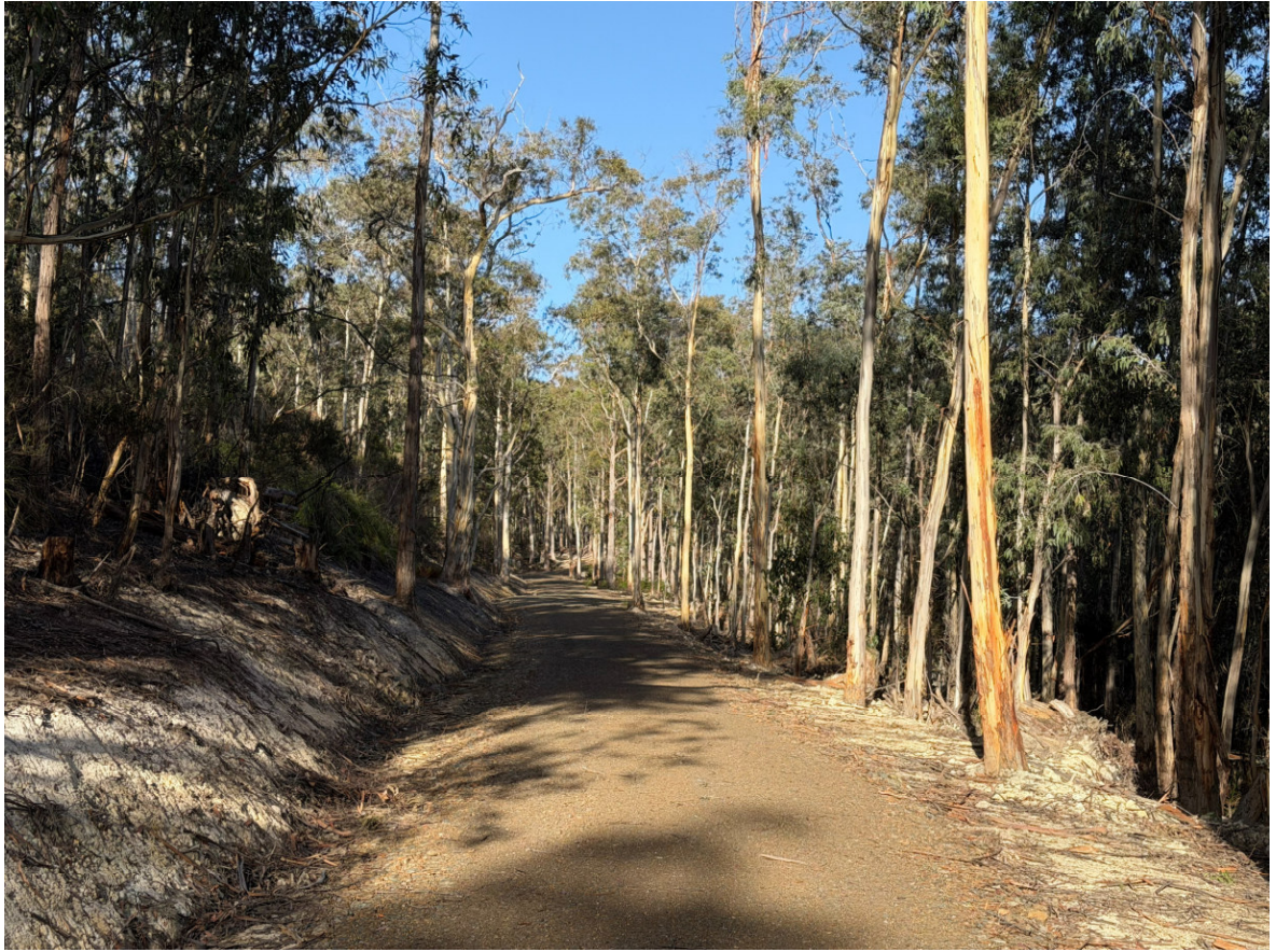
IMAGE 2: Completed driveway from property boundary to dwelling envelope
