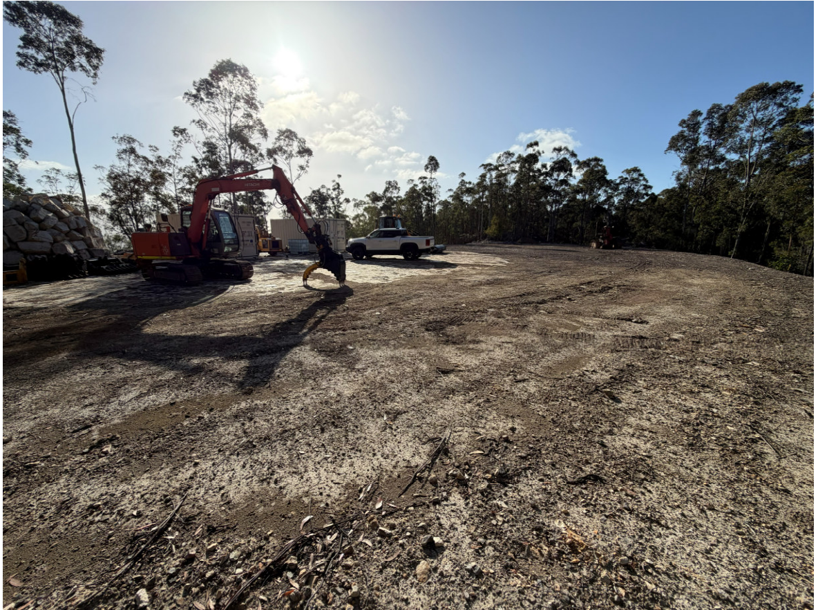
INSERT IMAGE 3: Completed earthworks at the dwelling envelope
