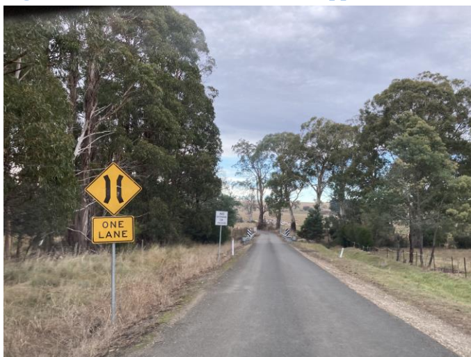
Figure 19 – Boomer Road Southern approach to Distillery Creek
