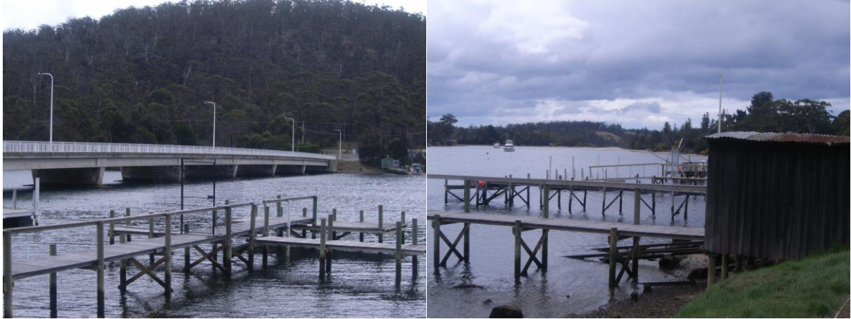
Bridge crossing the Prosser River and boat mooring facilities at Orford.
