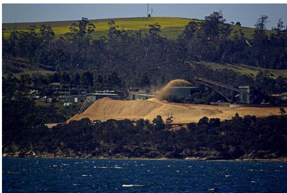
Former view looking east when the woodchipping facility was operational
