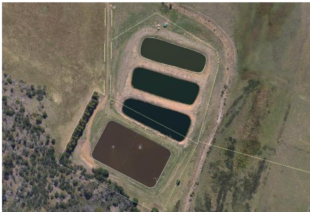
Figure 38-1: Orford Sewage Treatment Plant
