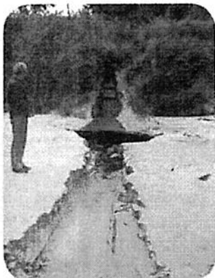
Figure 1.1: A bioretention swale for stormwater control at a residential development in the City of Hobart.
