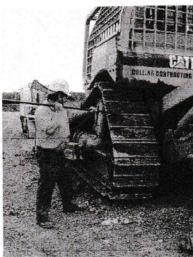
Chipping off compacted soil from tracks with a crowbar.
